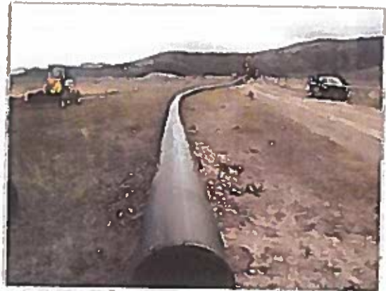
FIGURE 19 - HDPE BEFORE IT WAS PLACED
