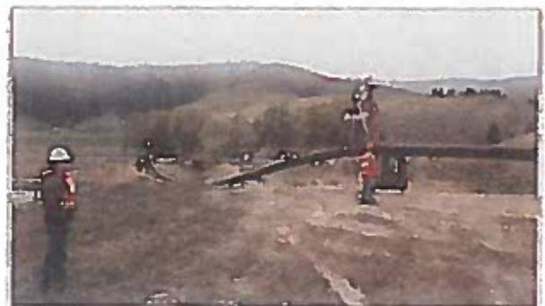
FIGURE 18 - PLACEMENT OF SIPHON PIPE
