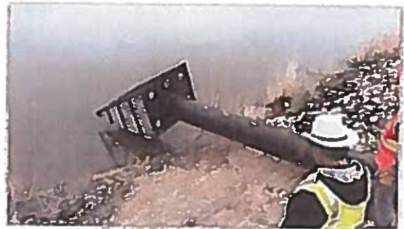
FIGURE 8 - INLET SCREEN ON SIPHON INTAKE
