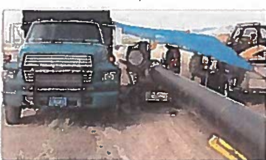
FIGURE 17 - FUSION OF HDPE PIPE
