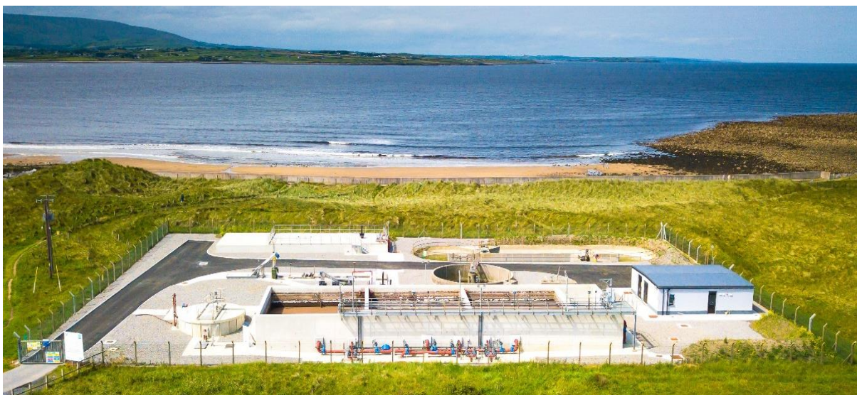
Figure 9: Strandhill waste water treatment plant
