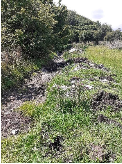
Figure 6: Drain with works, running along county boundary.
