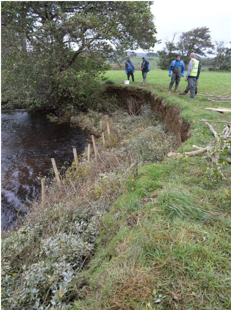
Figure 7: Example of brush soft engineering – Photo 1
