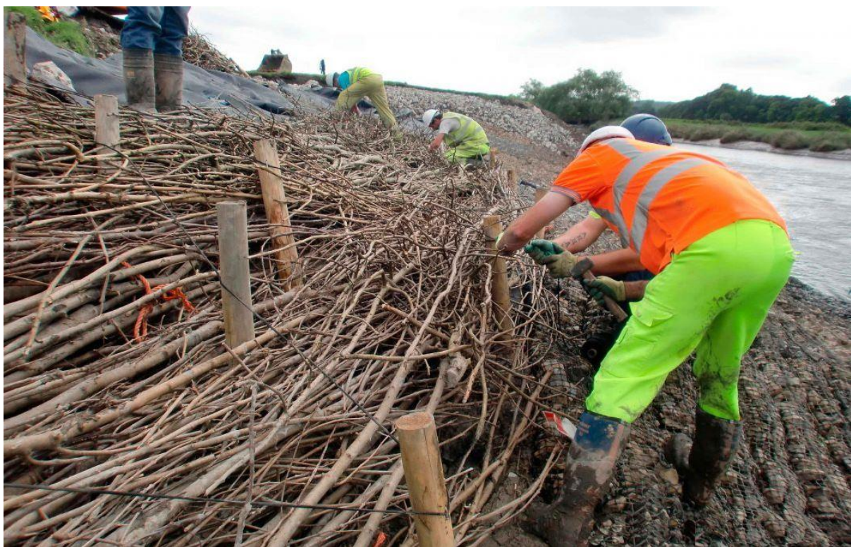
Figure 10: Example of brashwood fascine soft engineering works – Photo 2
