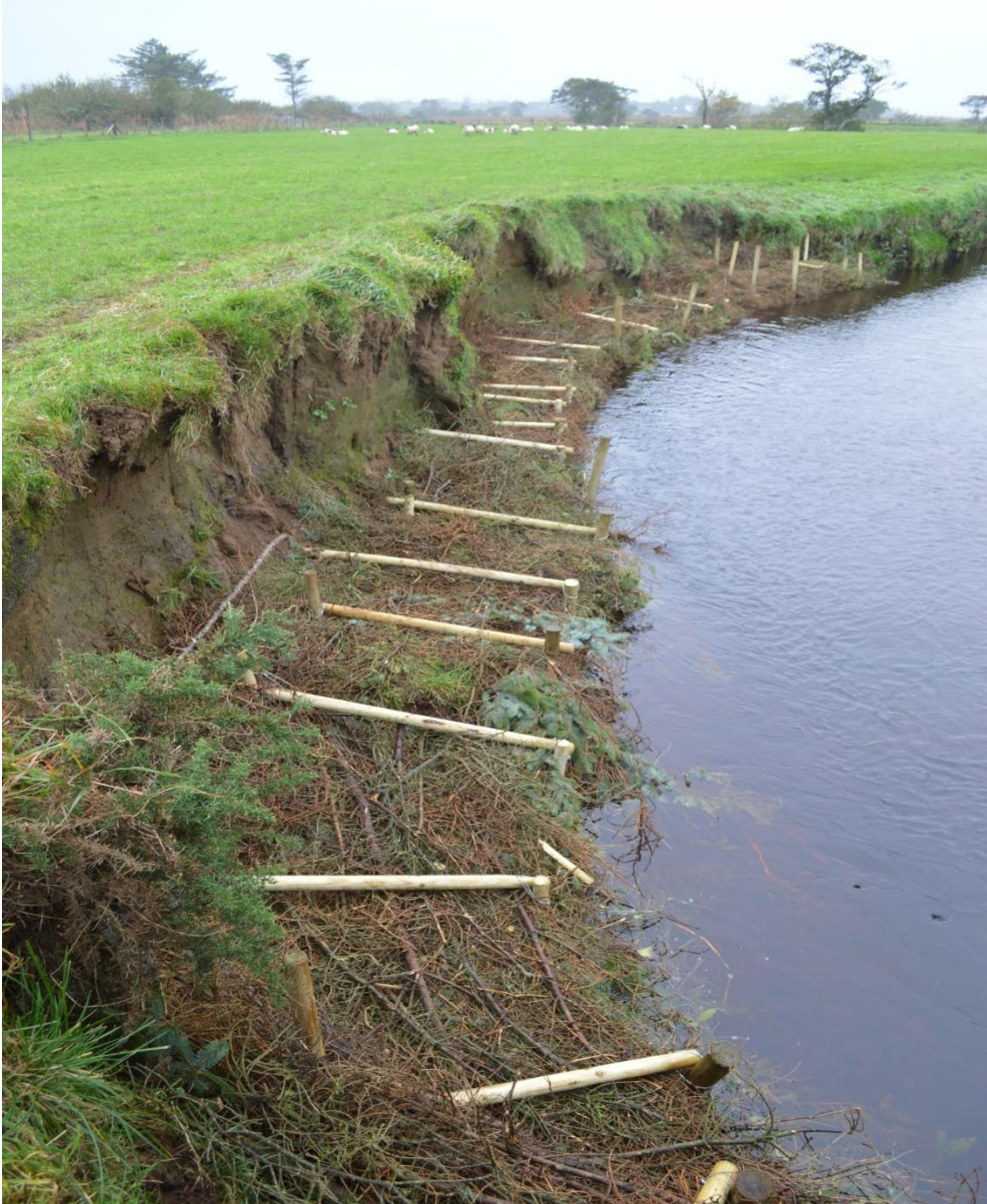
Figure 8: Example of brush soft engineering works – Photo 2
