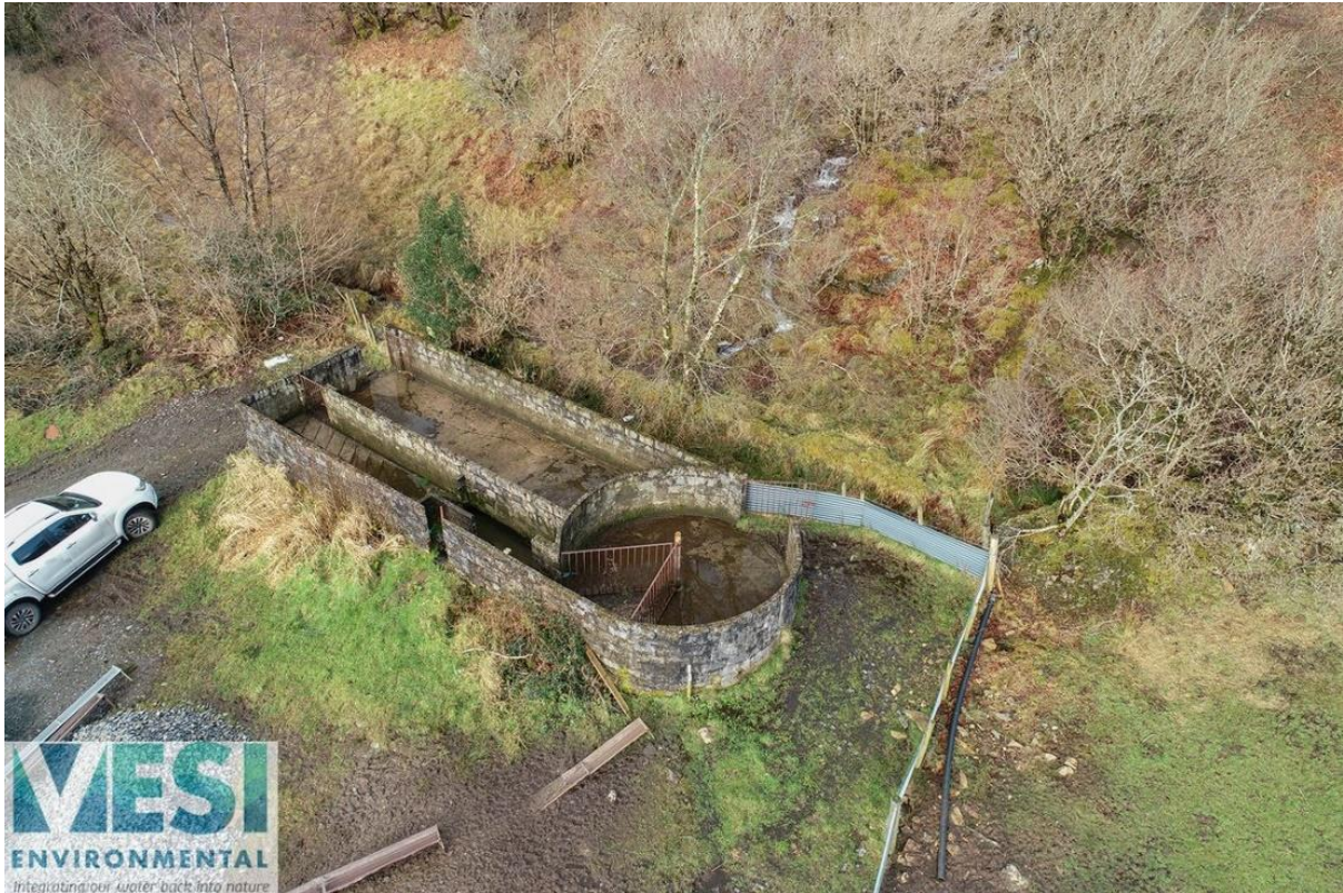
Figure 5: Sheep Dipping facility at Ballykerrigan.
