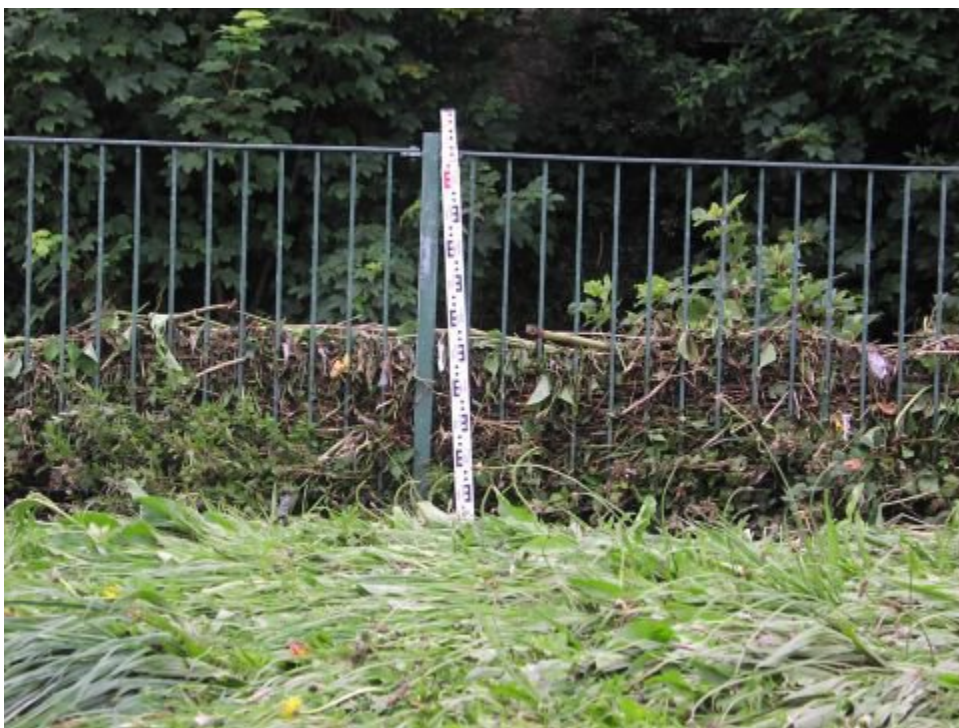
View showing depth of flood debris caught in railing along River Bride in Orchard Court (about 0.6m)
