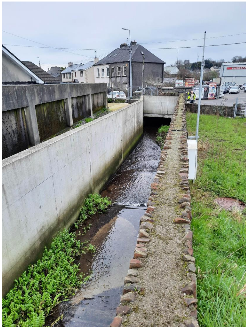
Photo: Townsend Street U-Channel & Culvert
