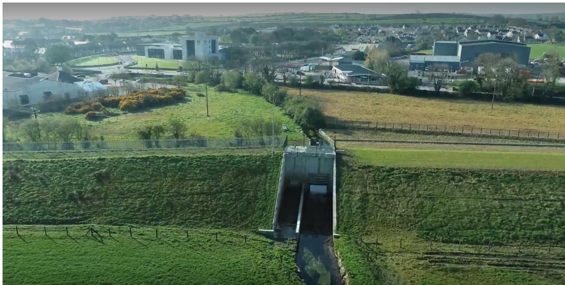
Photo: Clonakilty FRS – Flow Control Structure.
