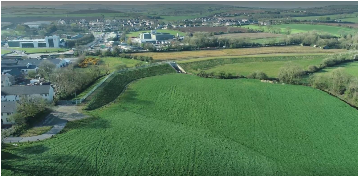
Photo: Clonakilty FRS – Flow Control Structure.
