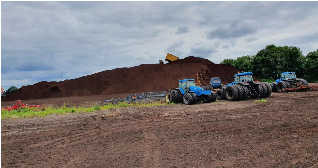
Photo 2: Large stockpile of milled peat at the loading area.
