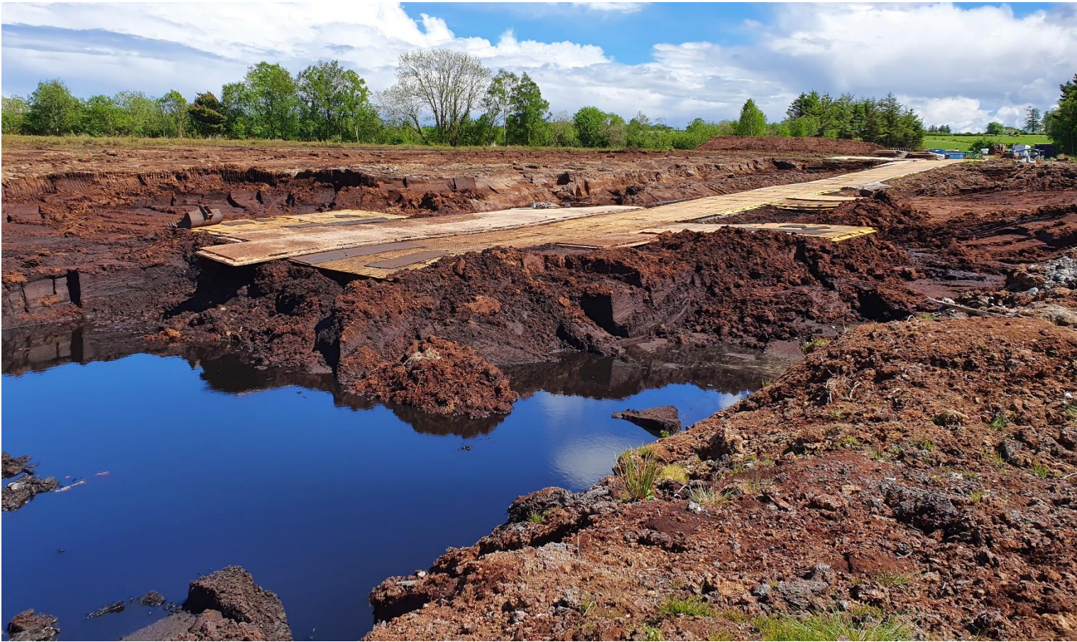
Photo 2: Temporary roadway constructed into excavated area.
