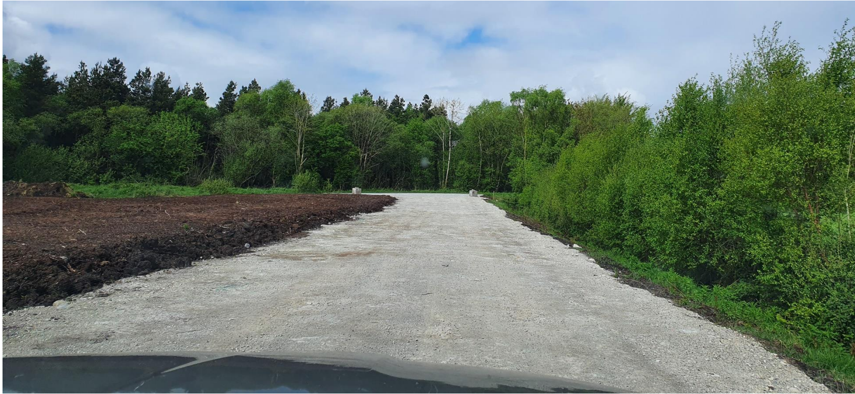
Photo 4: Newly constructed roadway into the peatland.
