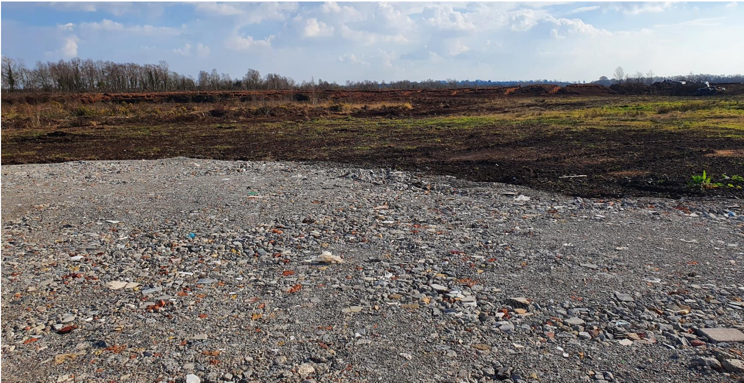
Photo 3: Recently constructed hardstanding with C&D fill noted.
