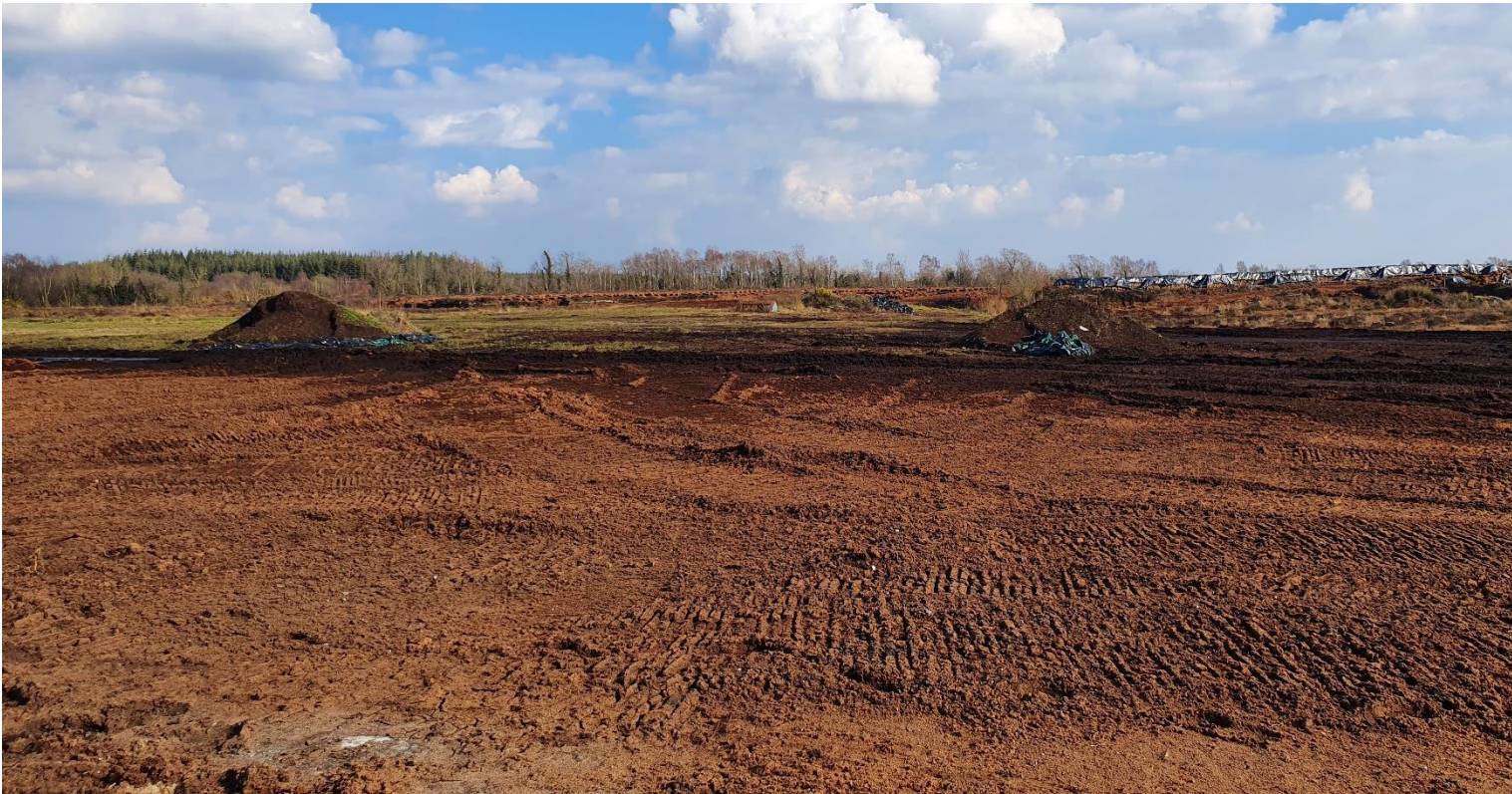
Photo 1: Recently excavated sod peat noted on the peatland.
