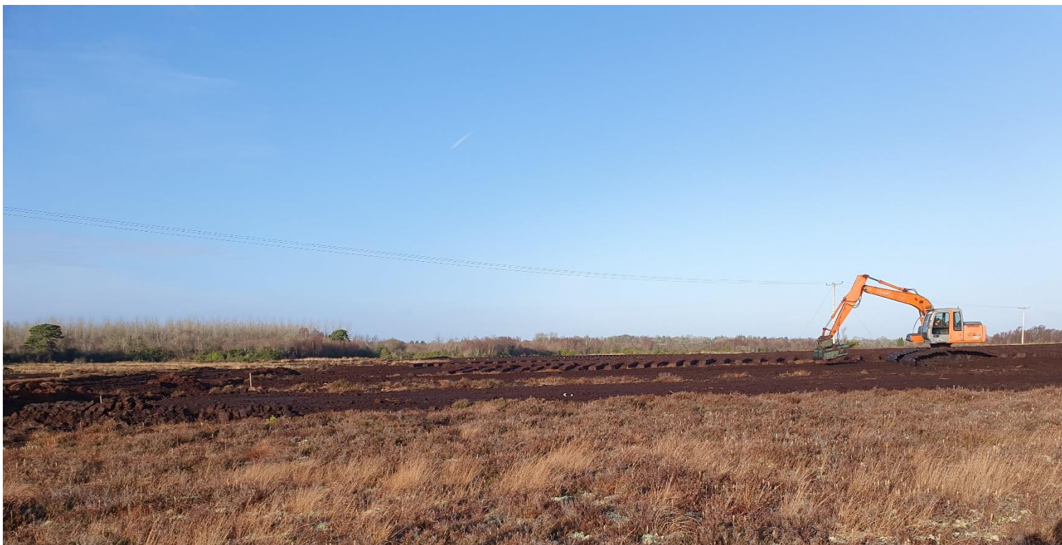
Photo 2: Excavator with large sod peat attachment noted on the peatland.
