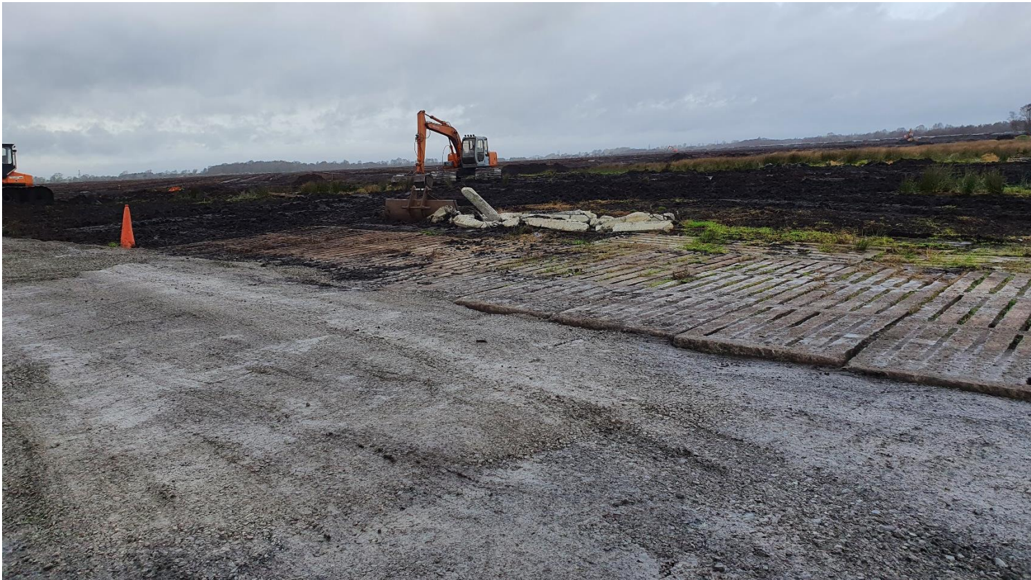
Photo 6: Purpose built roadway at loading area.
