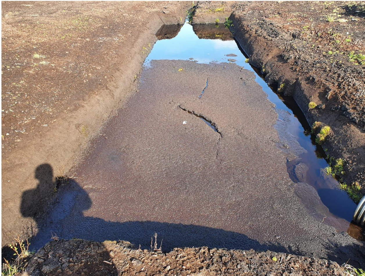
Photo 3: Silt pond for collection of silt from surface water.
