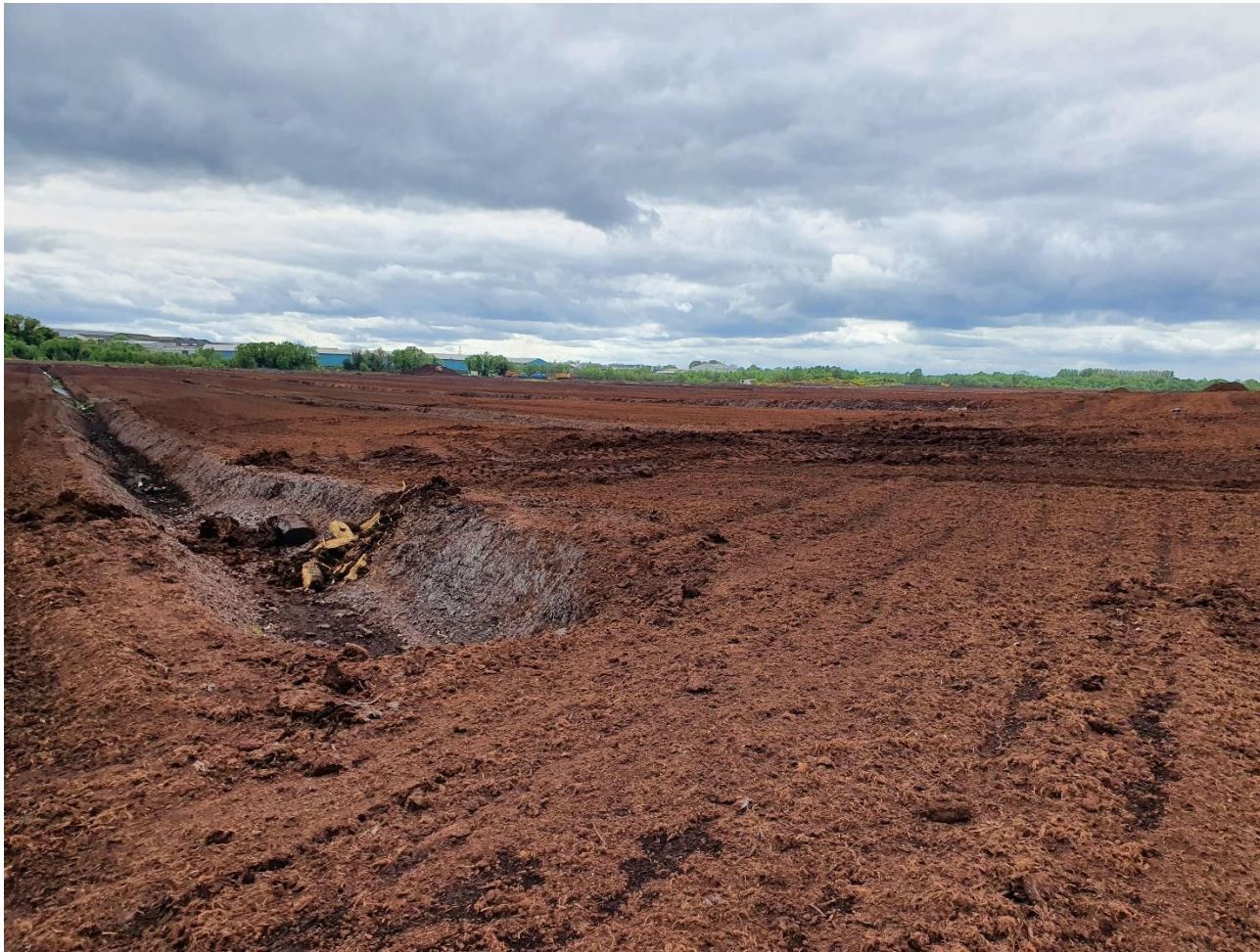
Photo 2: Recently tilled peat on peatland.
