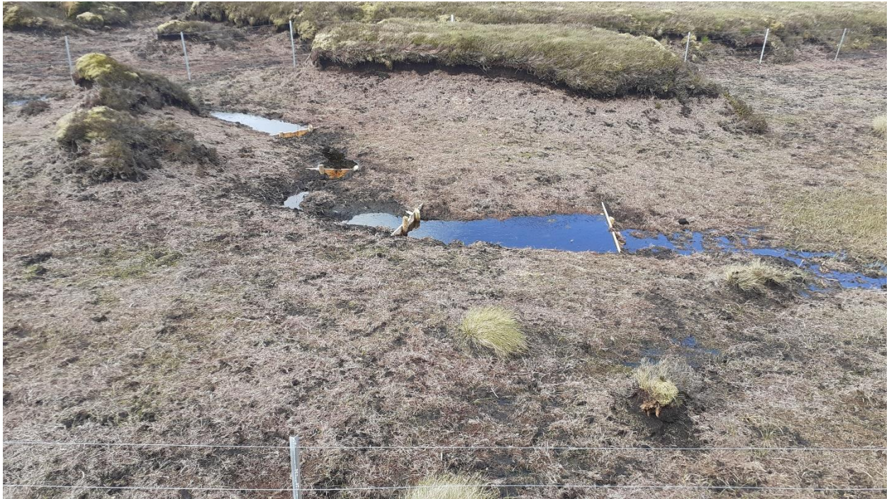
Photo 2 Example of bog restoration works in WMNP. Photo shows, fencing, reseeding and damming.
