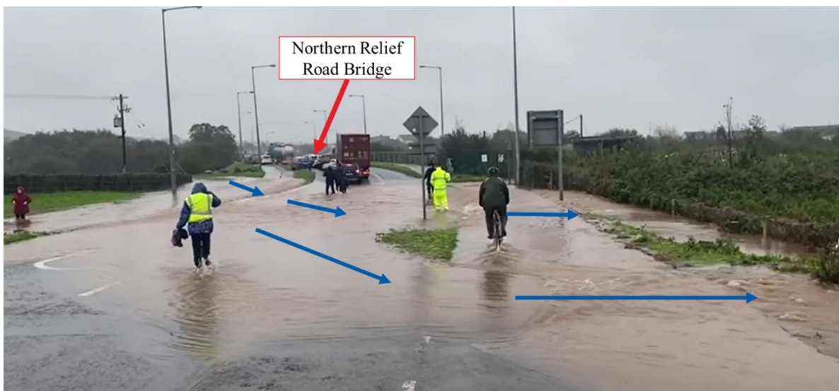
Figure 32: Water overtopping NRR West approach road
