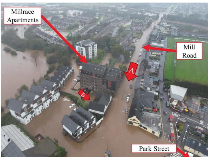
Figure 41: Flooding via Mill Road and the Millrace
