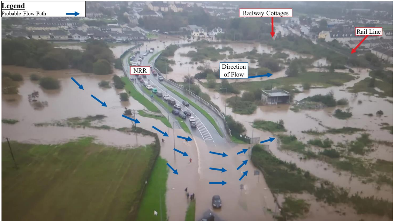
Figure 33: Water overtopping NRR West approach road (arial image)
