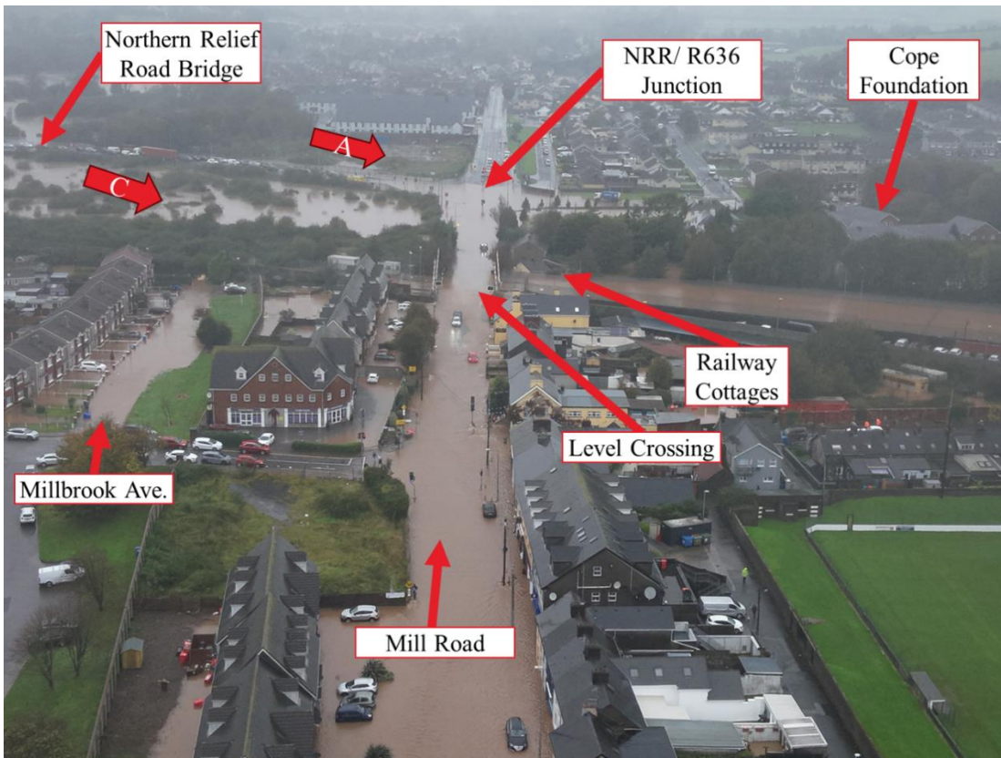
Figure 35: Aerial Image of Northern Relief Road/ Rail Line Level Crossing (Guileen Coast Guard)
