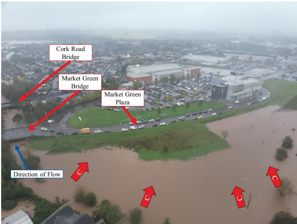
Figure 42: Flooding on Right Bank Upstream of Market Green Bridge
