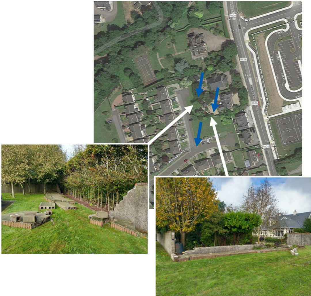
Figure 26: Boundary Walls Failed
