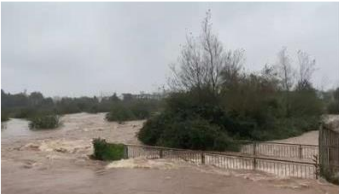
Figure 34: Bridge Downstream of NRR Bridge surcharged
