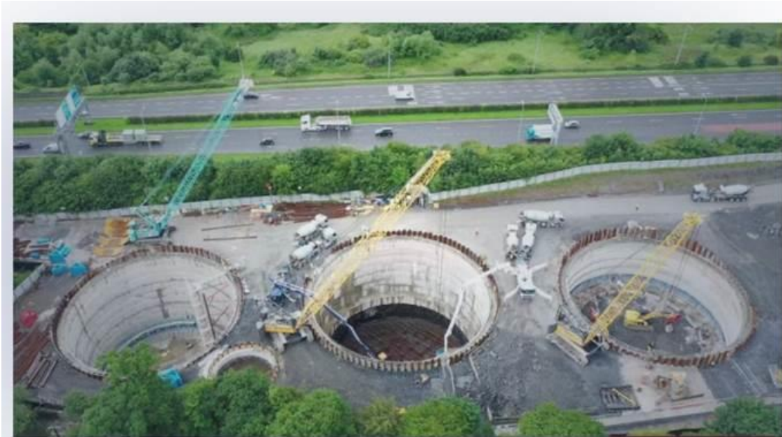
Blanchardstown 9c sewer storm tanks, Co. Dublin
