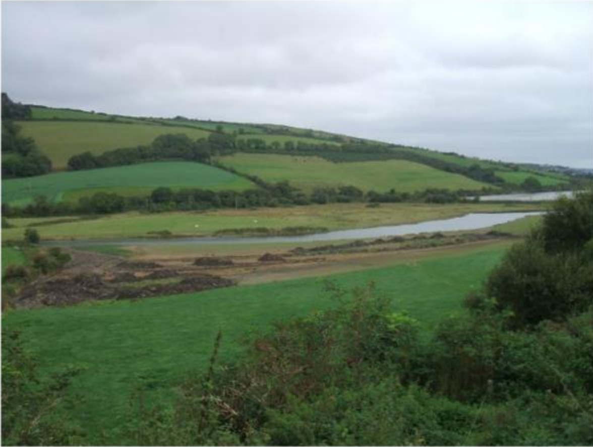
Example of Drainage work, claimed to be clearing old drains.
