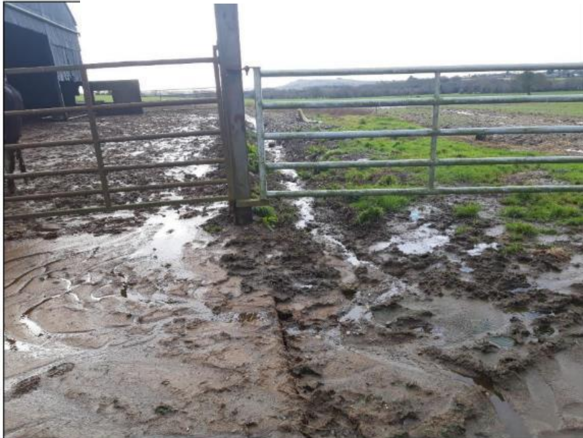
Photograph 1: Slurry & soiled Water not contained with farmyard
