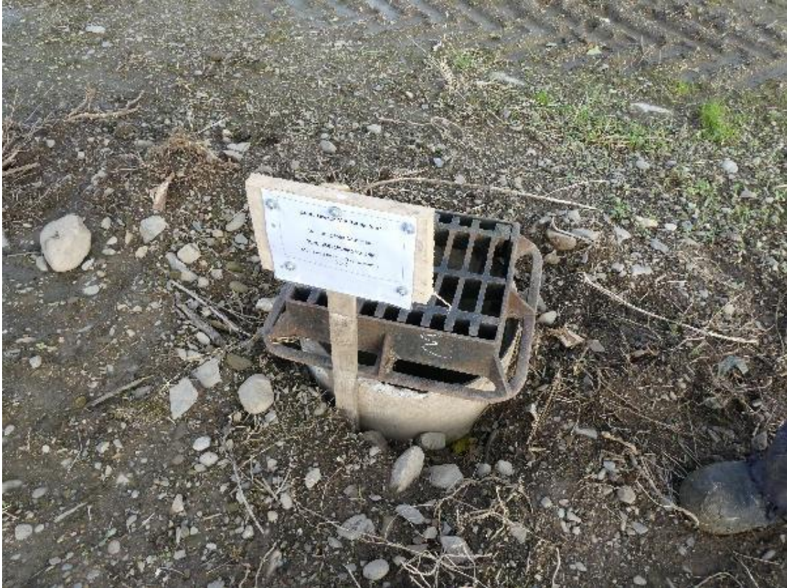
Photograph 3: ST-3 surface water emission point
