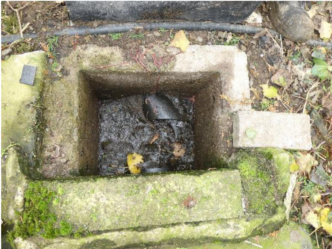
Photograph 4: ST-4 surface water emission point
