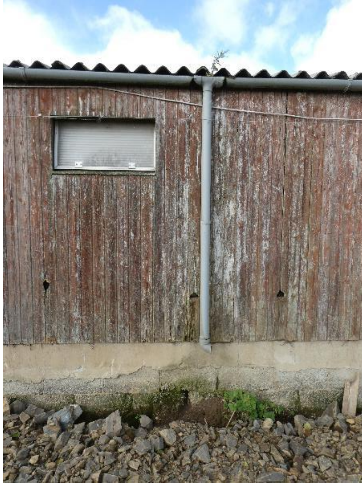
Photograph 1: Rainwater downpipe on animal housing unit
