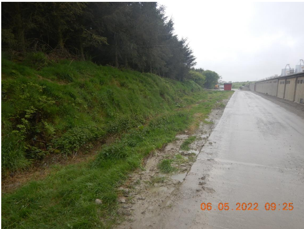
Photo 6; Photo of access road at licensed facilities.
