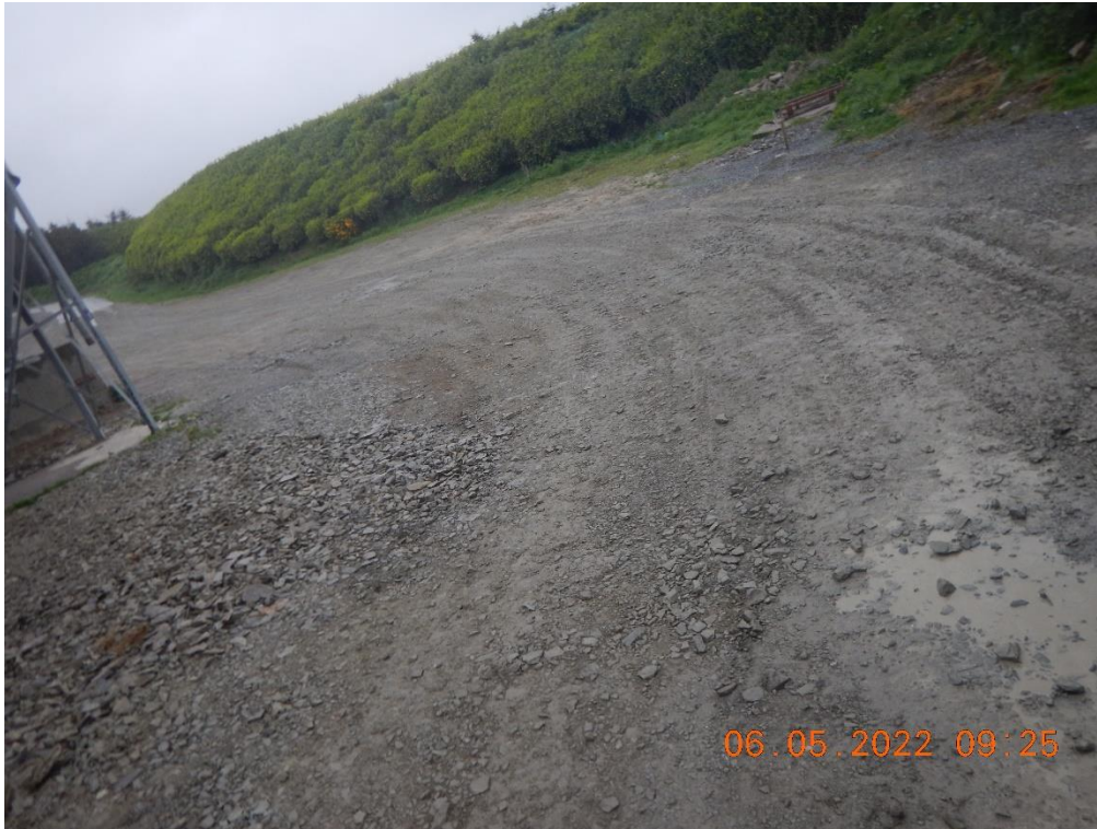
Photo 7; Photo of access road at licensed facilities.
