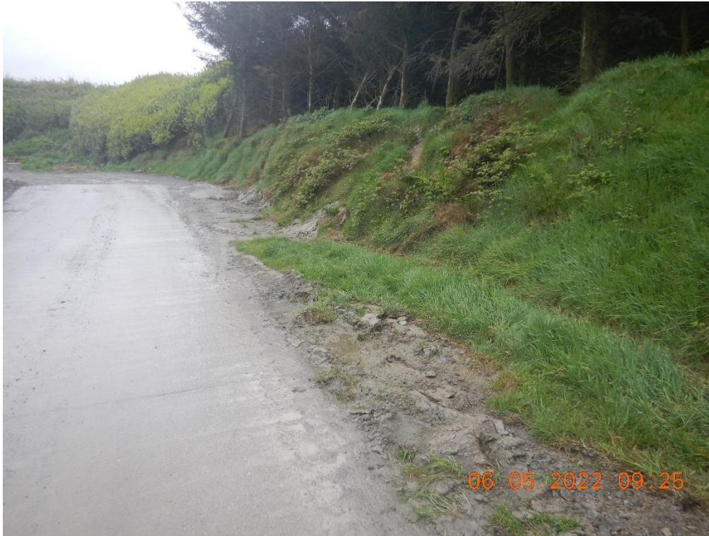
Photo 5; Photo of access road at licensed facilities.
