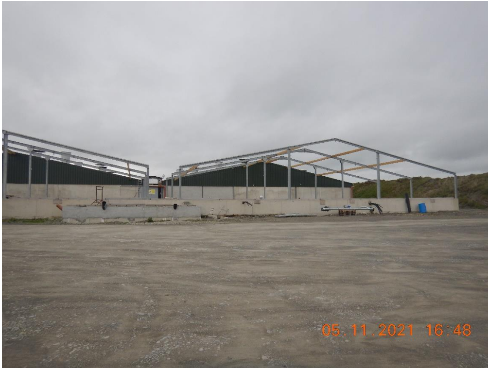
Photo 15; Additional sheds under construction.
