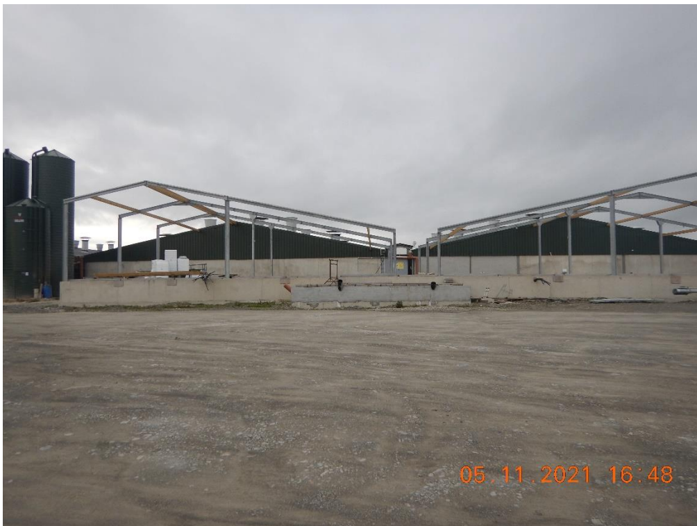
Photo 14; Additional sheds under construction.
