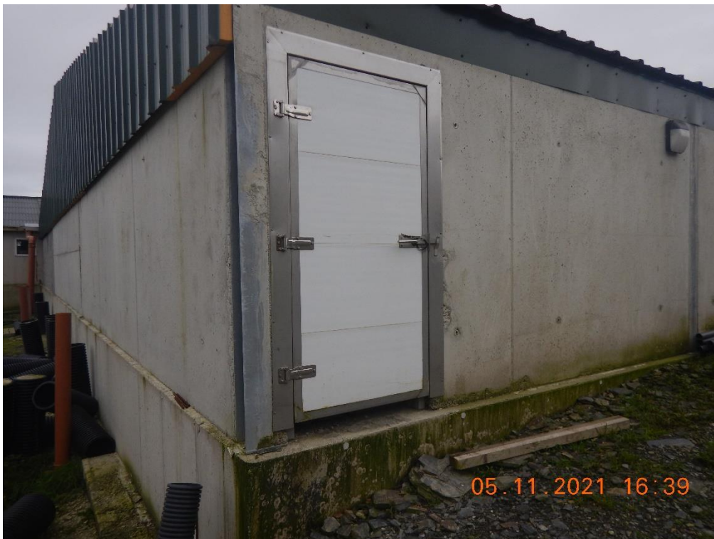
Photo 12; External door of pig house.
