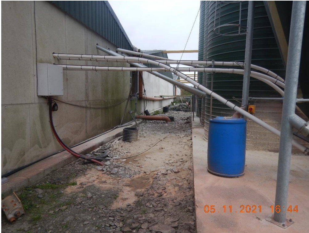
Photo 13; Unprotected ground adjacent to feed silos.
