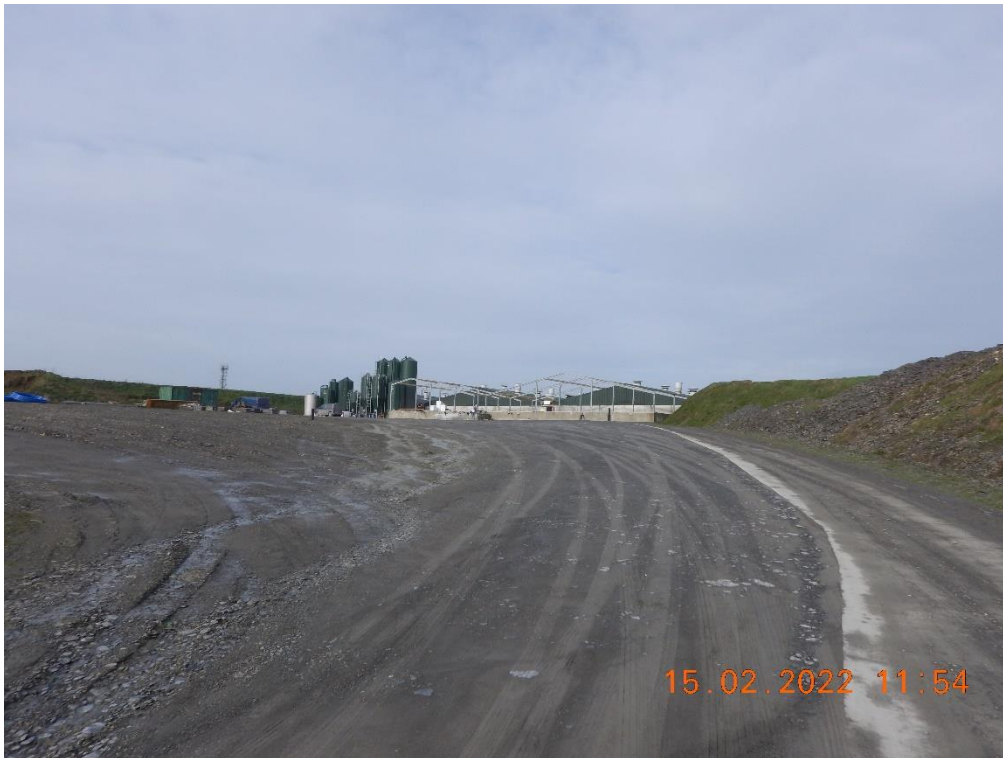
Photo 1; Photograph of facilities outwith licensed site boundary.
