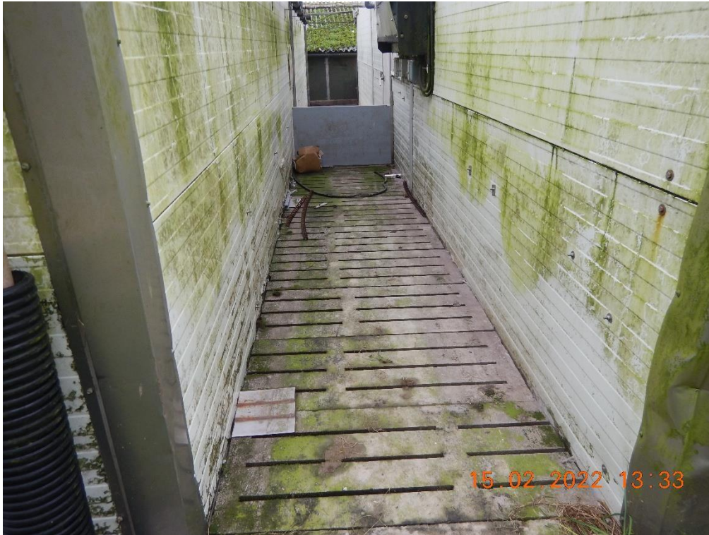
Photo 9; Photograph of uncovered tank.
