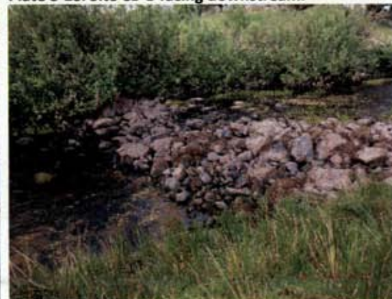
Plate 3-30: Example of boulder weir across river.
