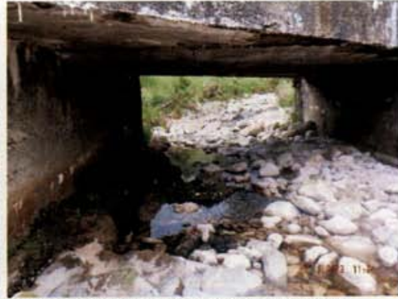
Plate 3-12: Bridge at site DB-4 facing upstream.
