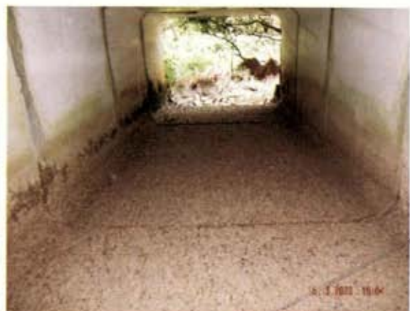
Plate 3-6: Dry box culvert upstream of site DB-2.
