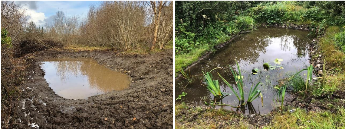
Figure 4 Pond installed by Cúlra Créafóige at discharge point of subsurface land drains in the Ray Catchment during construction, and 6 weeks later with some macrophyte planting (Iris, Nymphaea, Stratiotes, Caltha, Menyanthes)
