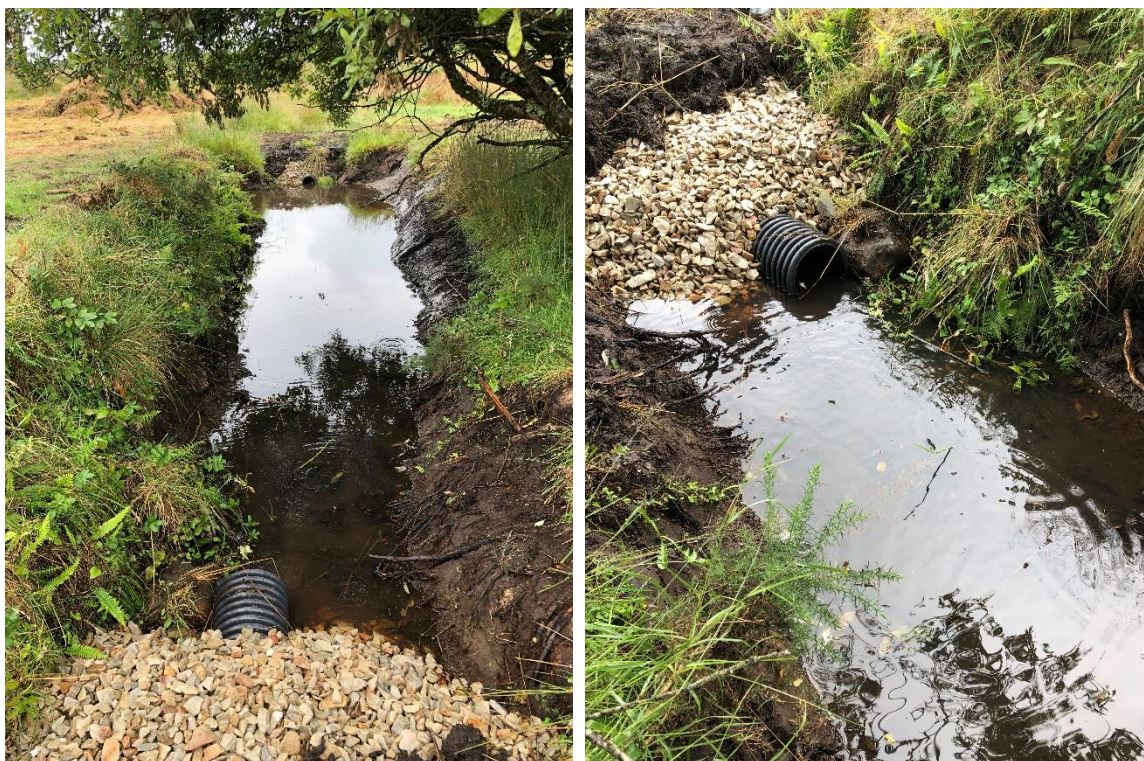
Figure 5 Drainage ditch with settlement/biodiversity pond construction (now fenced) showing culvert pipe and angular quartzite stone.
