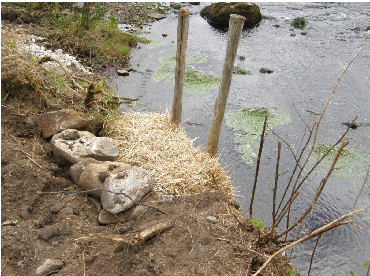
Figure 5 Use of straw bales to dam ditch outfalls during works
