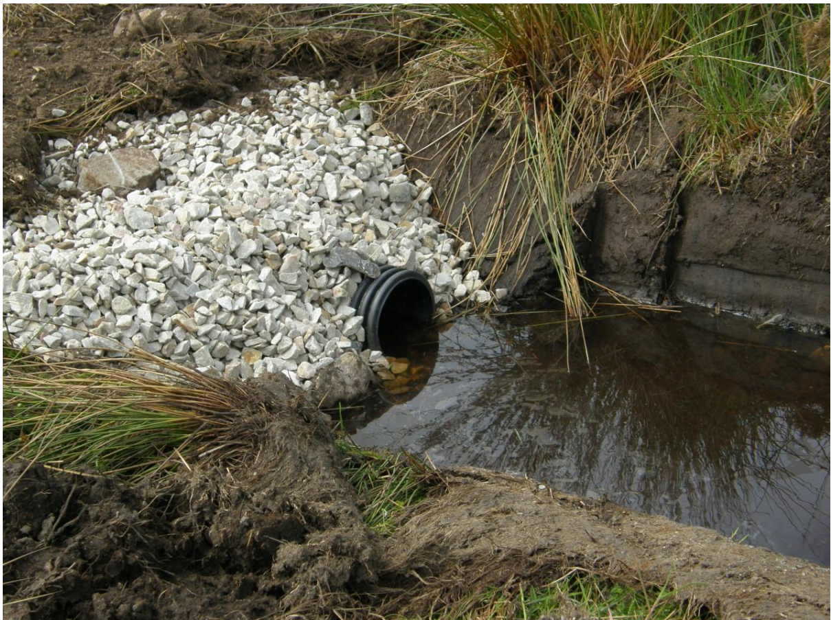
Figure 4 Culvert construction using clean quartzite stone
