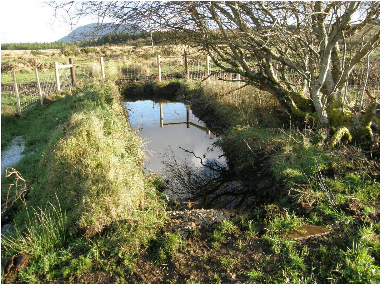
Figure 6 Deepening and widening of drains to create settlement sumps at the outfall
