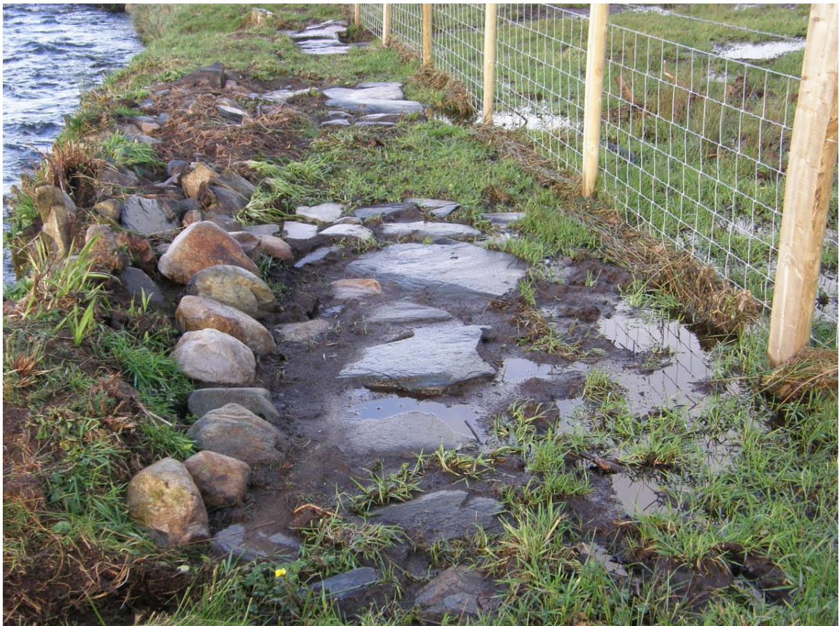
Figure 8 Stone protection on damaged bank surfaces in the riparian buffer strip
