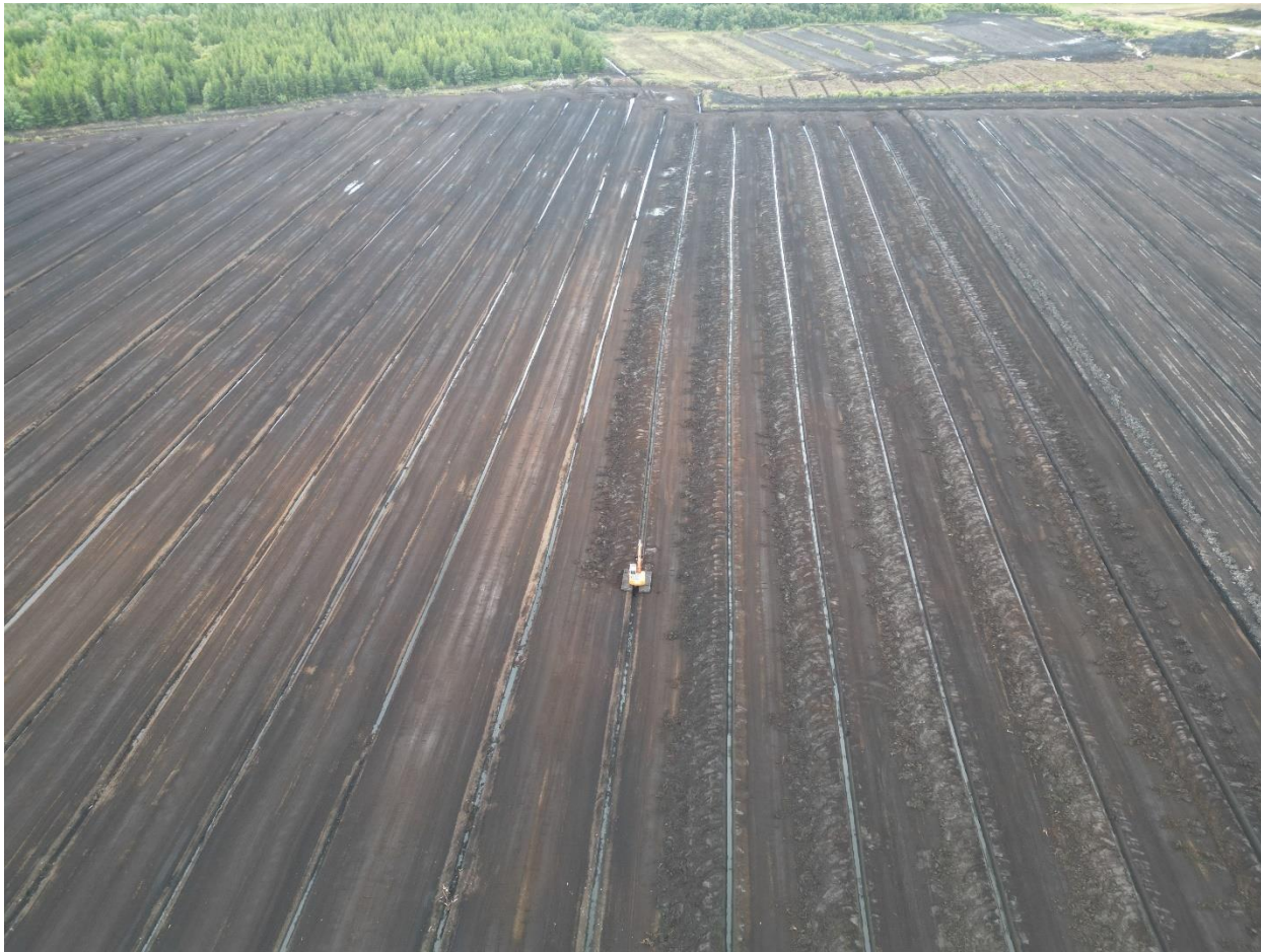
Photo 1: Excavator carrying out drainage works on the peatland.
