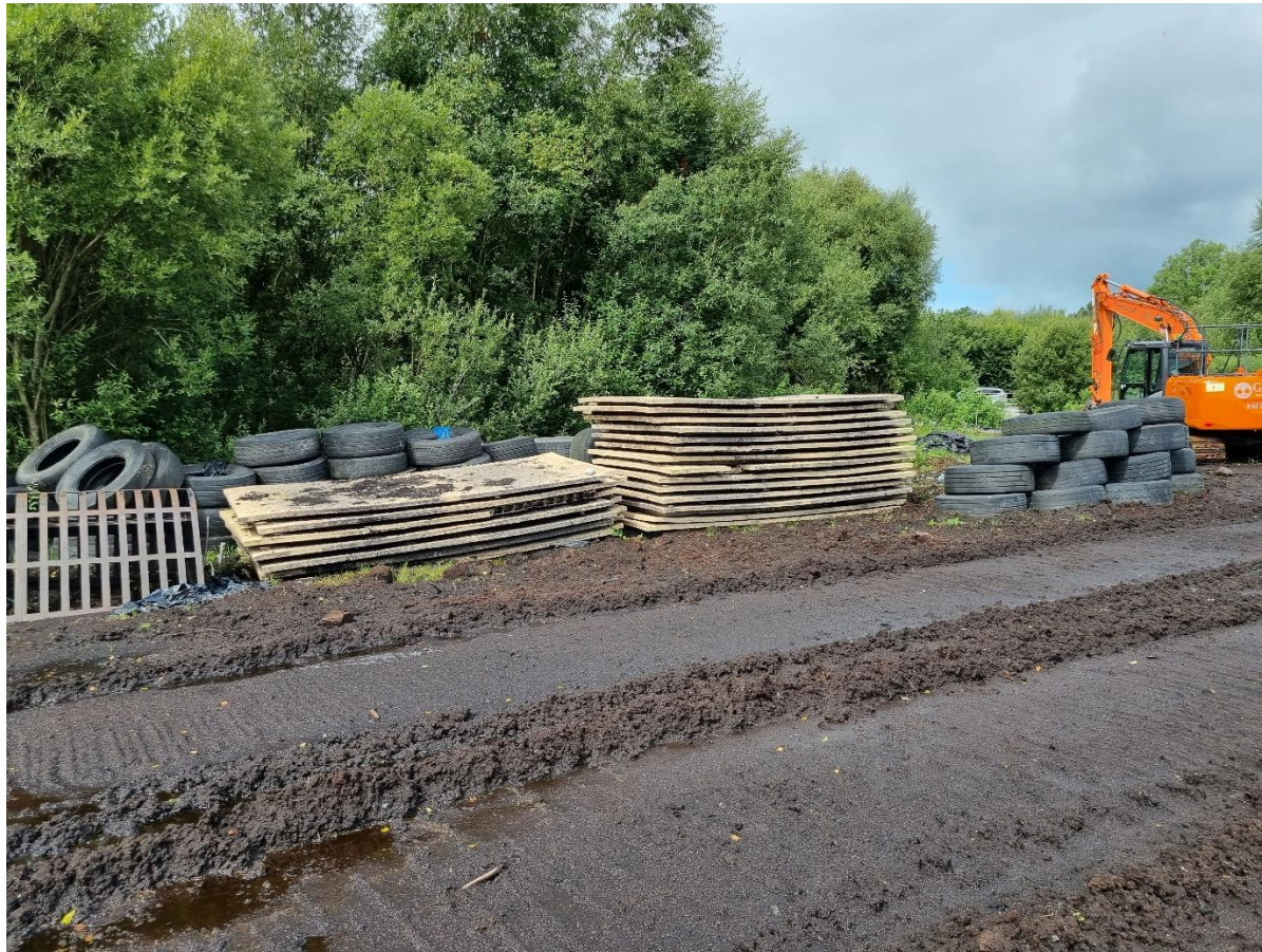
Photo 5: Temporary road structures noted at the loading area.
