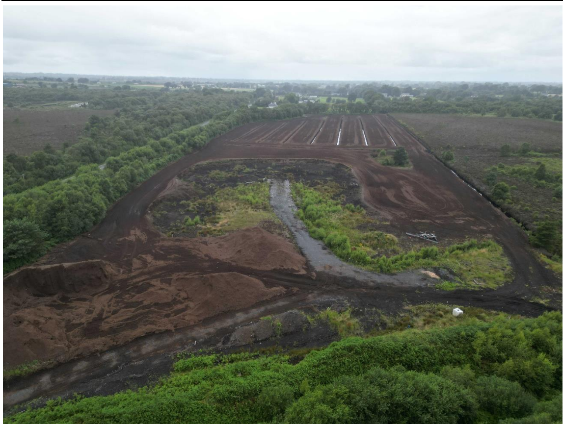
Photo 3 – Western part of the site with stockpile of milled peat.
