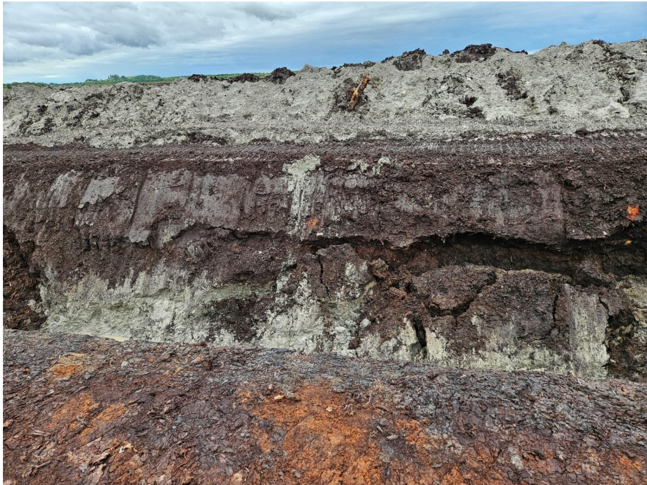
Photo 4: Photo showing slippage in some of the drains on the peatland.
