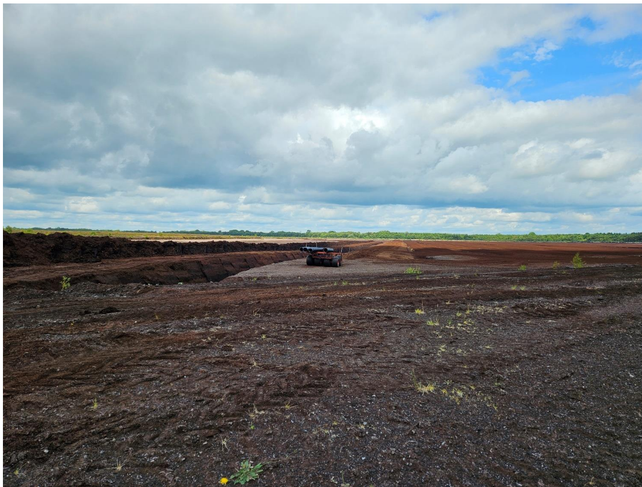
Photo 3: Photo of ongoing drainage works at the peatland.
