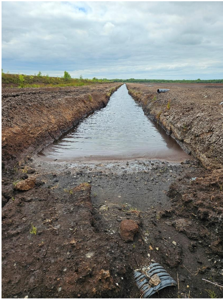
Photos 7 & 8: Drainage network with significant sediment build up noted at the South Eastern corner of the peatland.
