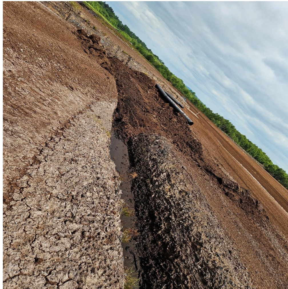
Photo 5: Drainage works noted at the Northern part of the peatland.
