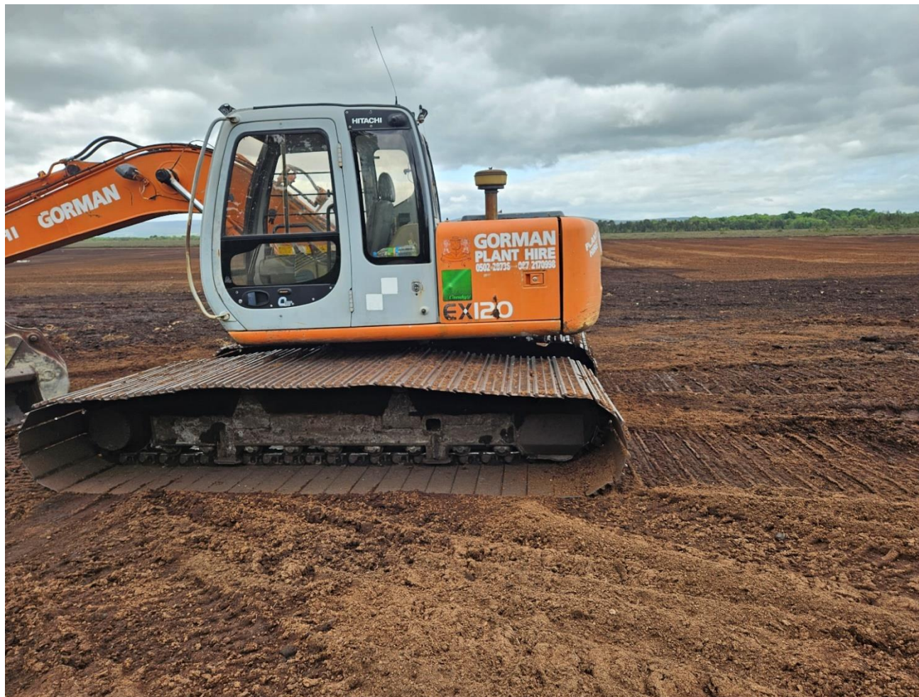
Photo 5: Photo showing excavator with 'Gorman Plant Hire' noted.
