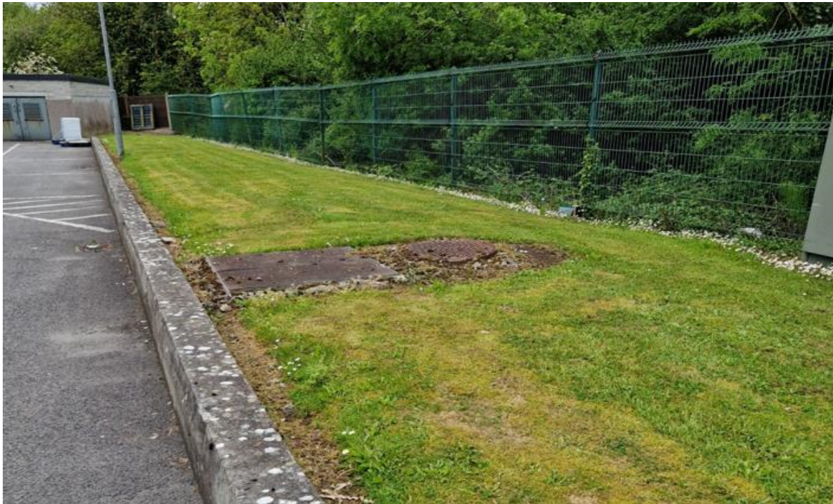
Figure 17 SWO to the rear of Dunnes Stores to be assessed for misconnections due to impacted water quality downstream.
