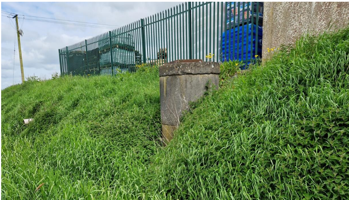
Figure 9 Manhole which needs assessing for overflows near Connaught Road.
