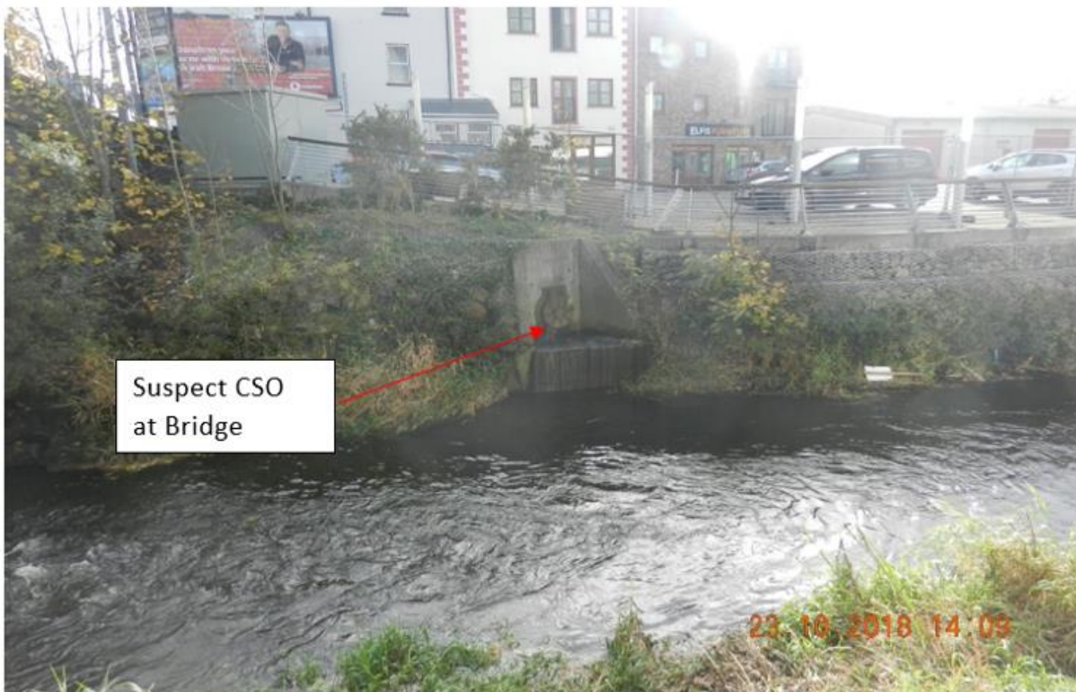
FIGURE 5 Suspect CSO at Little Water Street which is activated in moderate rain conditions.
