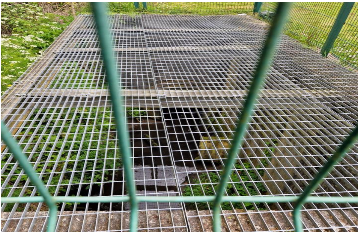
Figure 16 SWO to the rear of Dunnes Stores
