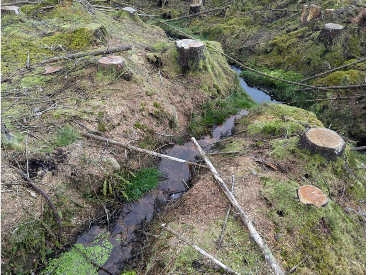
Image 11: RWC intercepting AZ with no mitigation. Signs of sediment release from nearby crossing point.
