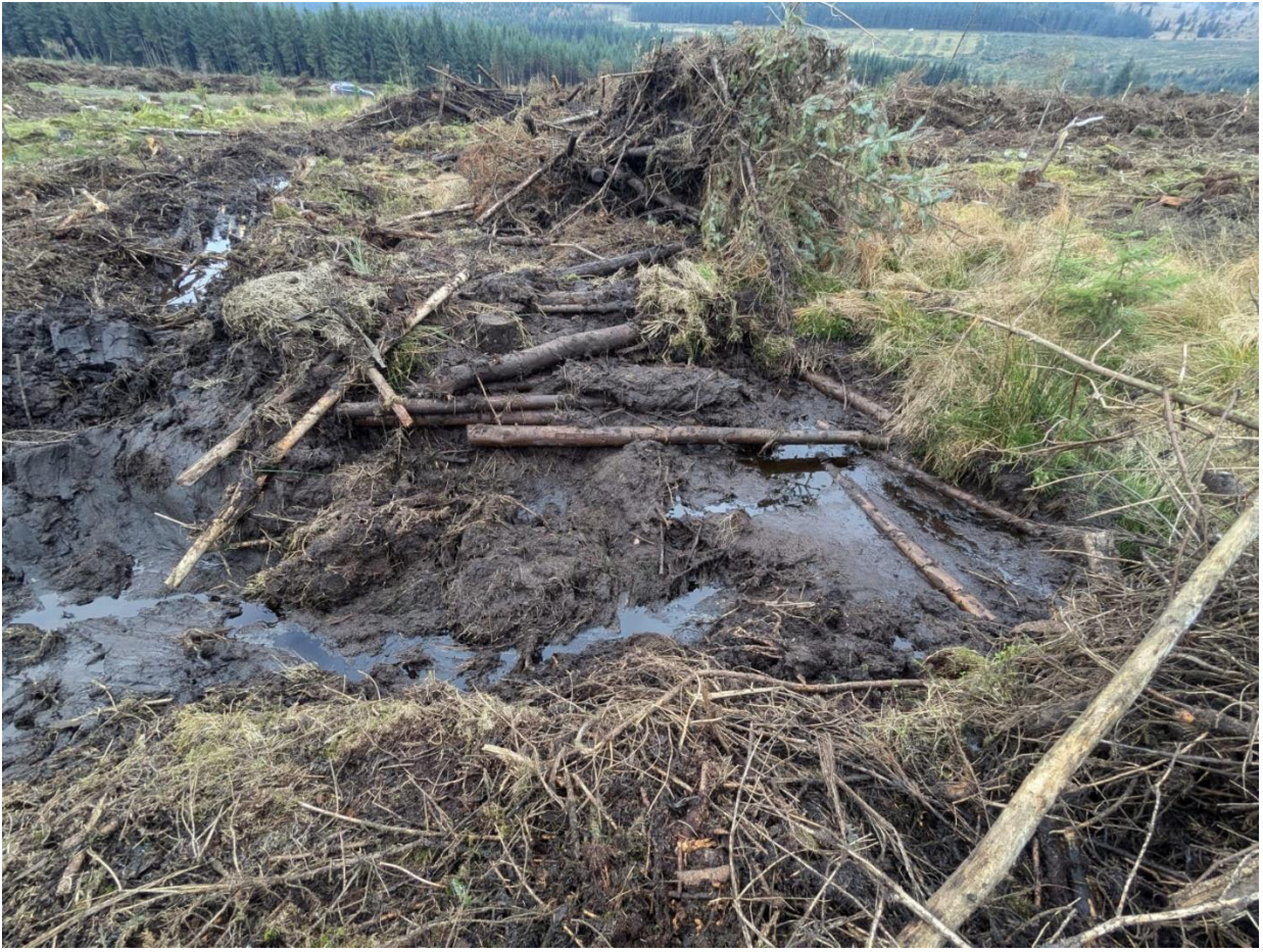
Image 5: RWC crossing at hotspot. Significant mobilisation of sediment.
