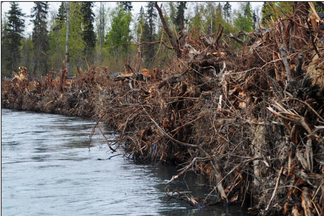
Plate 9. example of LWD use in erosion management.
