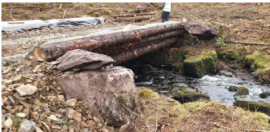
Figure 16. Temporary bridge.
