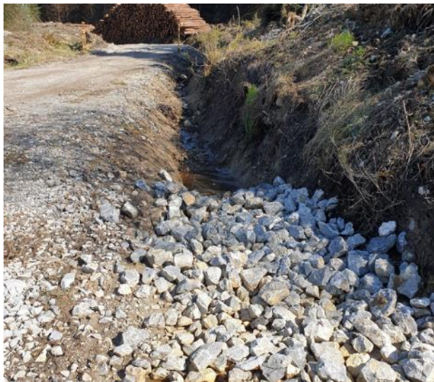
Figure 13. 3" or 4" clean washed stone placed in roadside drain.
