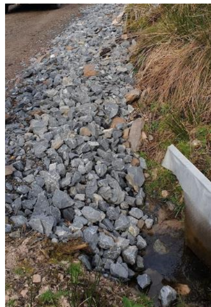
Figure 14. 3" or 4" clean washed stone placed in roadside drain with geotextile silt trap on the outflow.
