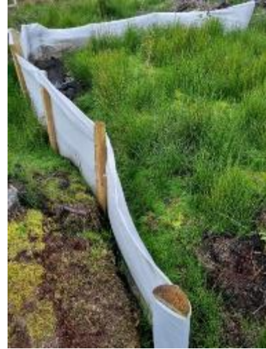
Figure 23. Silt curtain where the protected hotspot is vegetating over.
