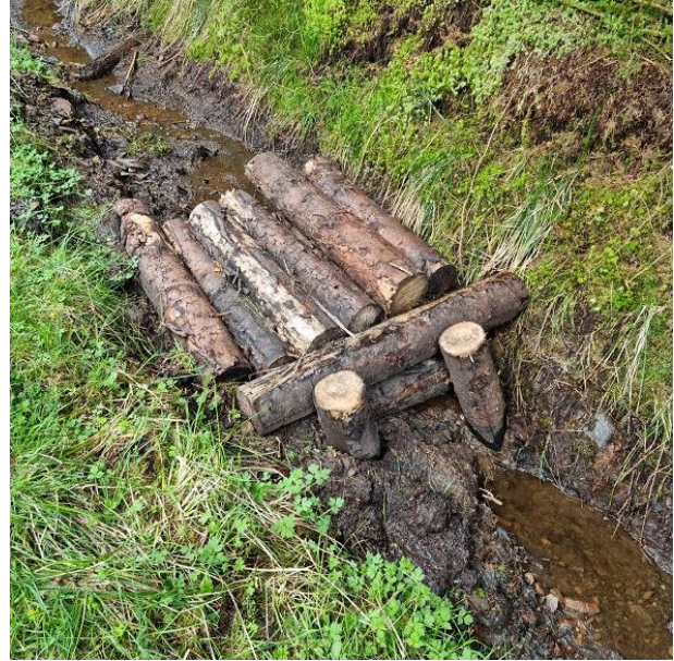
Figure 25 – Log / leaky dam located in a roadside drain, this will 'green up' or vegetate.
