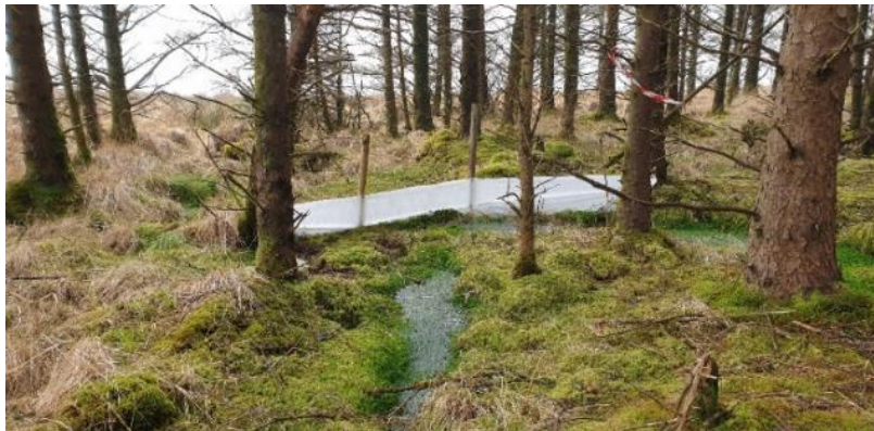
Figure 18. Silt curtain used to contain surface water siltation.
