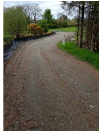
Figure 12. Another example of a roadside silt curtain.
