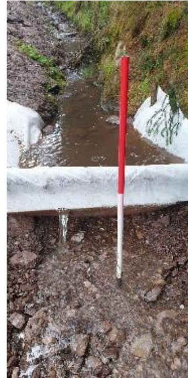
Figure 21. Newly installed functioning silt trap suitable for site with impenetrable substrate.
